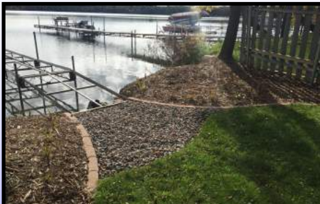
Roos Lakeshore Restoration & Washout Repair
