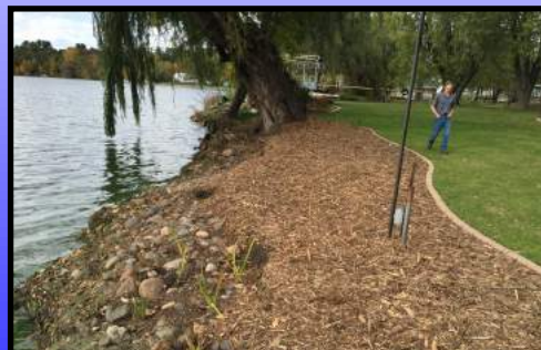
Lind Lakeshore Restoration & Vegetated Swale
