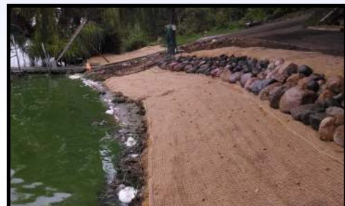
Hammer Lakeshore Restoration & Stormwater Diversion
