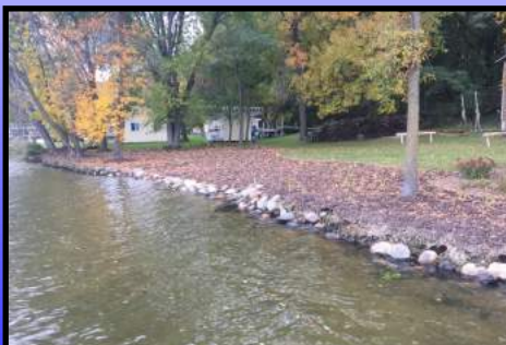
Hage Lakeshore Restoration & Washout Repair
