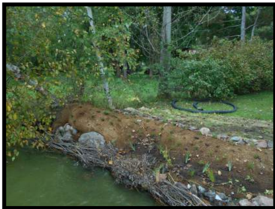
Small "ice heaves" were left in place to help control rain water runoff.
