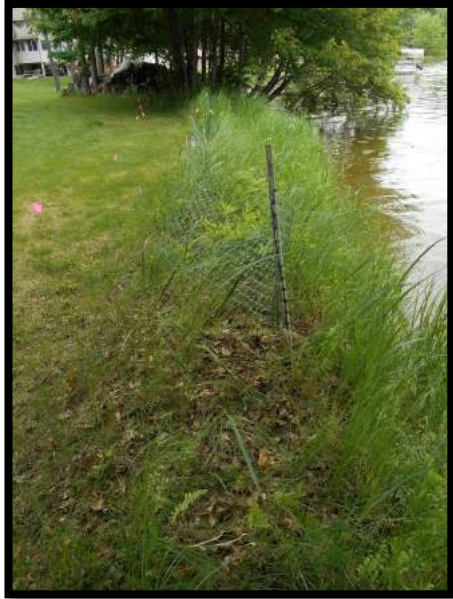
If native plants were present on site, like these sedges, they were saved and incorporated into projects.
